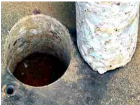
No Positive Side Vapor Barrier
